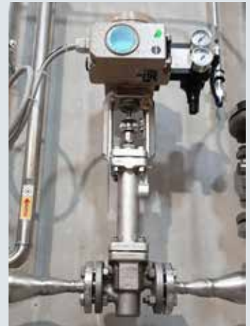
Hydrogen control by SAMSON Type 3241-7 Globe Valves with bellows seal.
